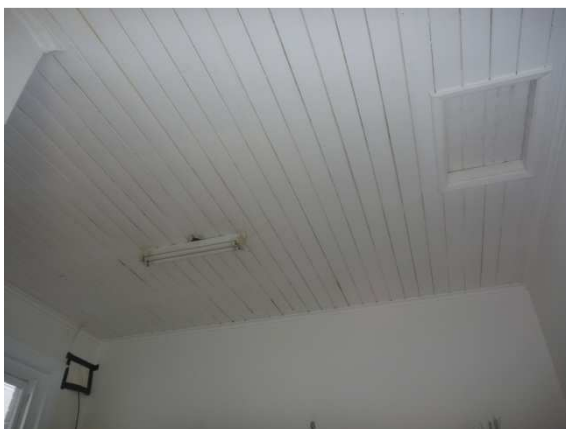
Timber ceiling in rear wing. Note: no cornices
