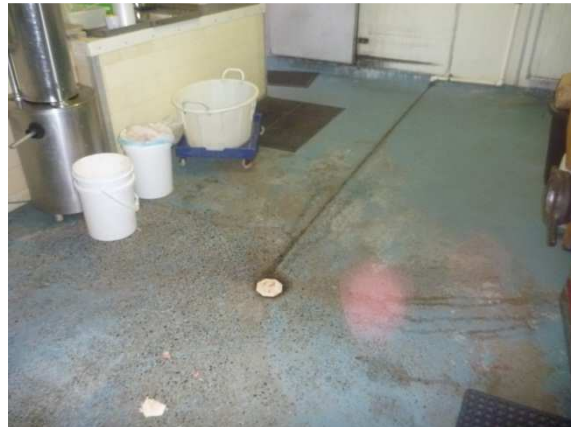
Sloped concrete floor leading to one drainage outlet in the 'boning room'.
