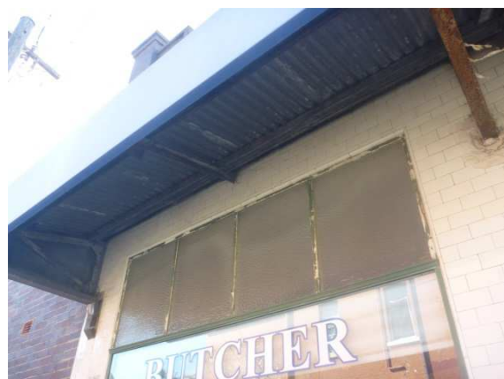
Original awning and window opening. However, window may have been replaced.
