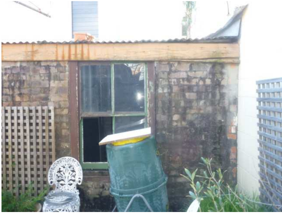
Southern elevation of rear garage structure.
