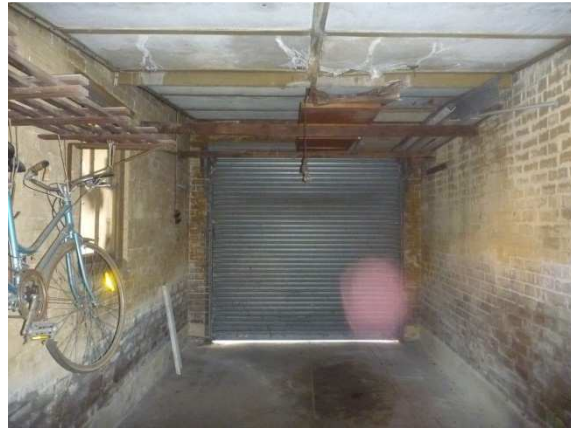
Internal view of the garage structure (facing west).
