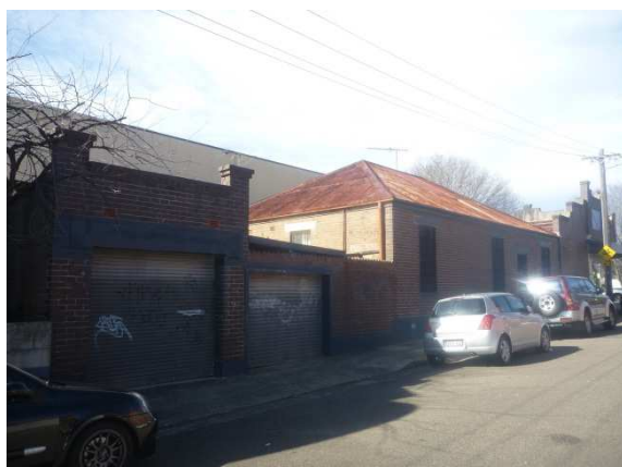
North Street elevation showing shopfront, residence and garage structure.
