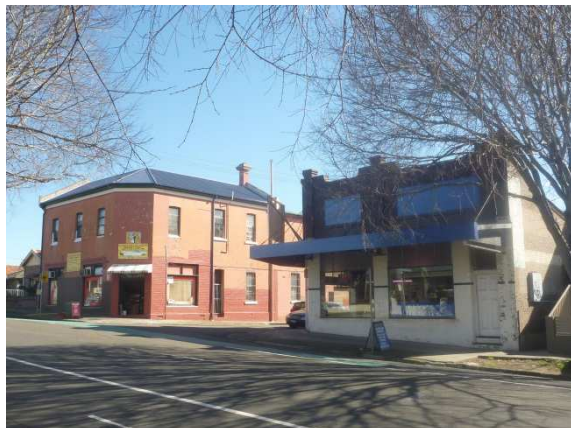
Allen Street relationship with No. 81 Allen Street opposite the subject building.
