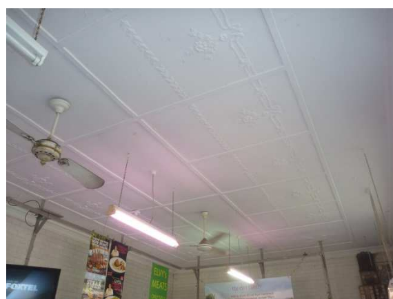
Decorative plaster ceiling in the shopfront.
