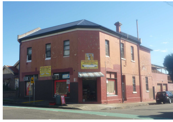
81 Allen Street (cnr North Street)
