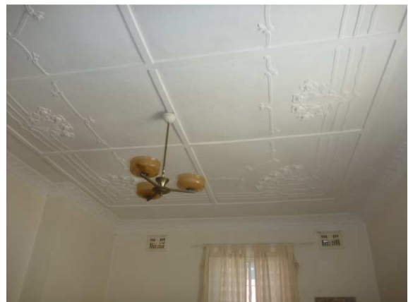
Decorative plaster ceiling and cornices in a bedroom.
