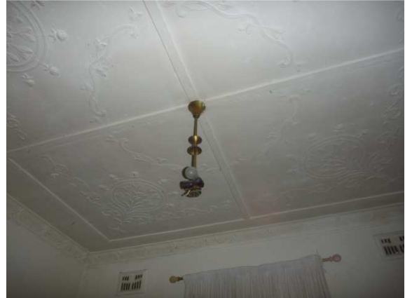
Decorative plaster ceiling and cornices in the living room.
